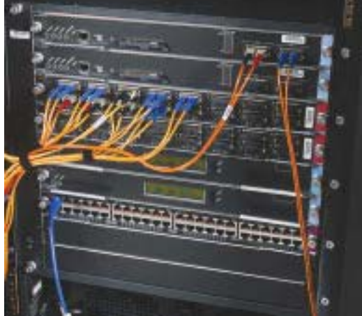
Switches from the Cisco Catalyst 6500 family, like this one, are at the heart of Altera's LANs.
